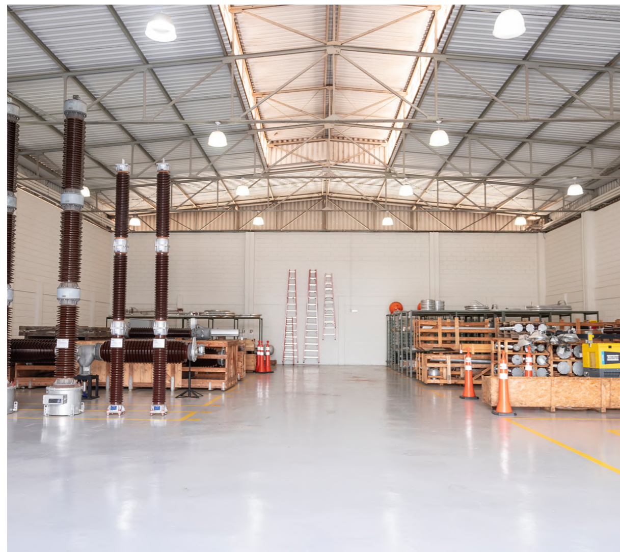
Maintenance base warehouse in Uberlandia, Brazil.
