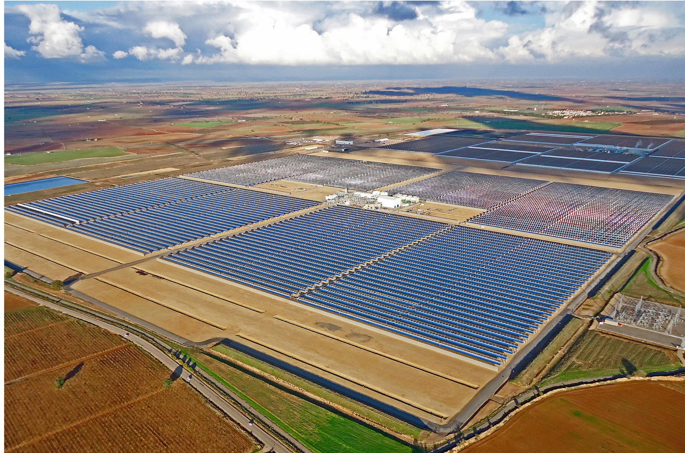
Solar Thermal Power Plant, Aste. Spain.
