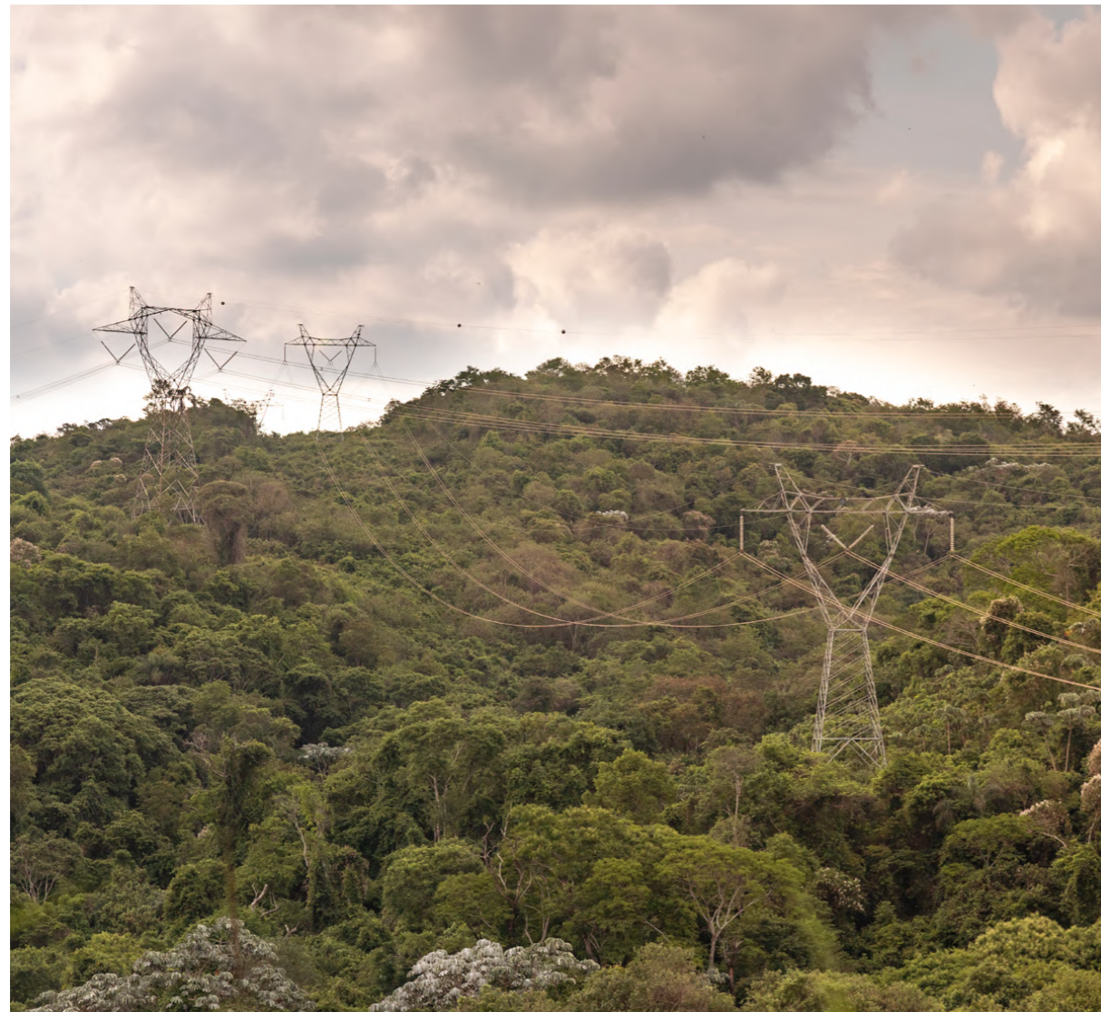
Cantareira transmission line, Brazil.
