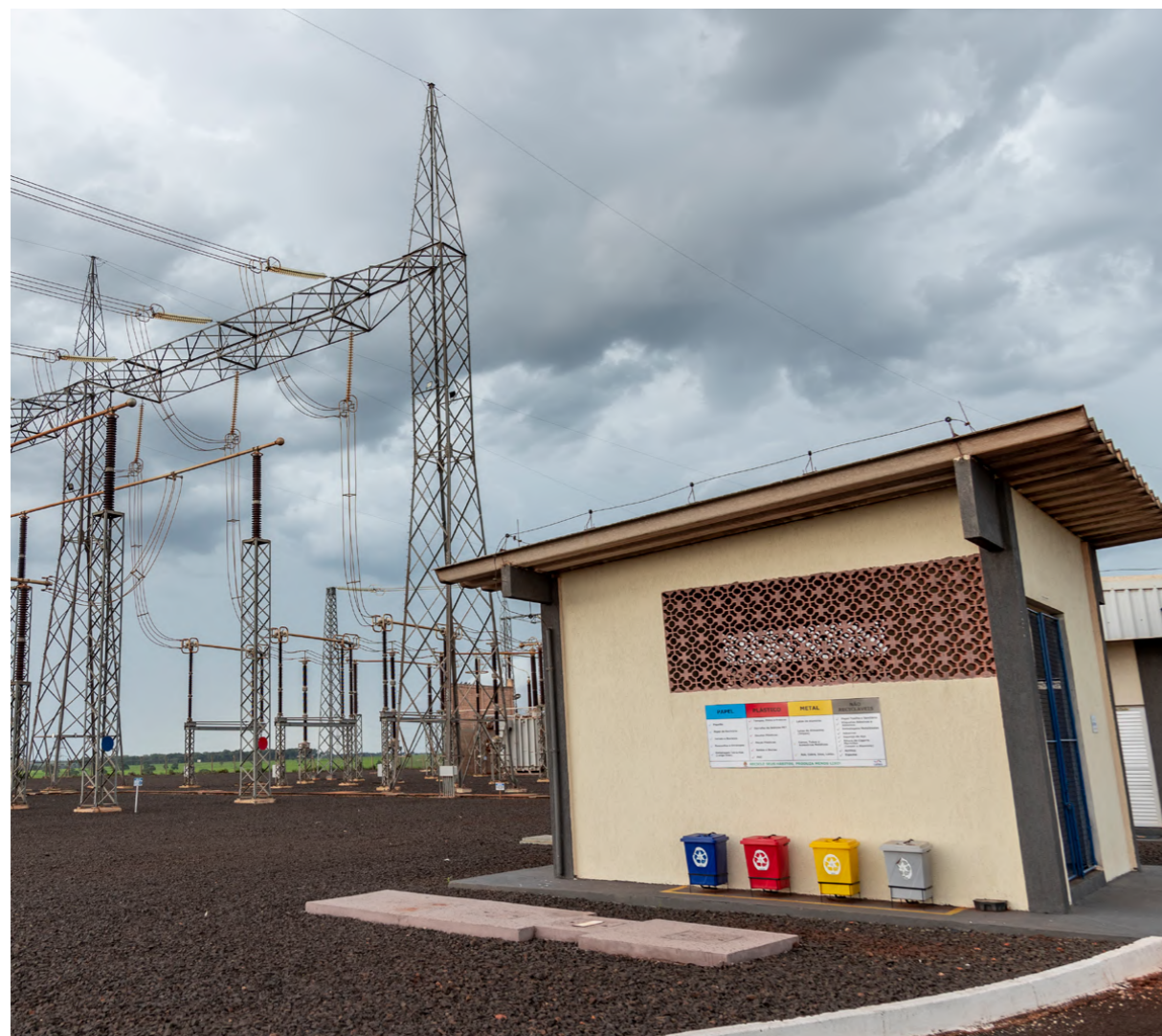
Waste segregation at the Itaguaçu substation of the Coqueiros transmission line.
