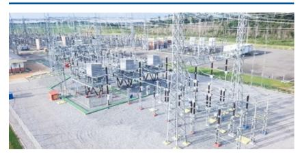
Also in 2017, reinforcement work began at Pedras Transmissora de Energia (PTE), with the installation of a third bank of 345-138 kV 3x133 MVA autotransformers in the Venda das Pedras Substation.
