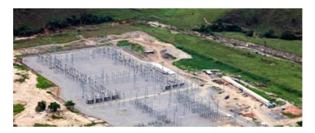
Some of the reinforcement projects that were implemented during the year deserve a special mention. In January 2017, the Reinforcement of the Linha de Transmissão Corumbá (LTC) became commercially operational, with the installation of a 230 kV bar reactor and associated modules at the Corumbá 2 Substation. The function of this Reinforcement is to assist in voltage
